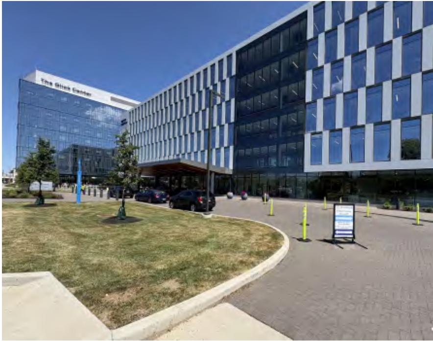
Main Entry Drive
