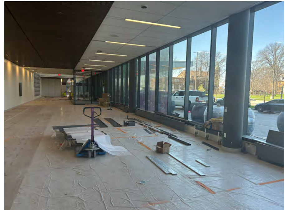
Ground Floor Public Lobby
