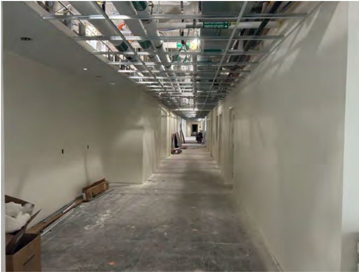
2 nd Floor Ceiling Grid
