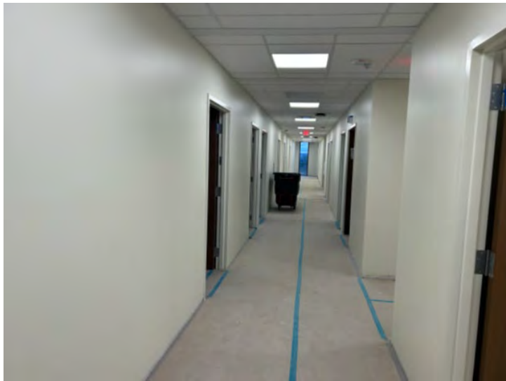
5 th Floor Final Paint
