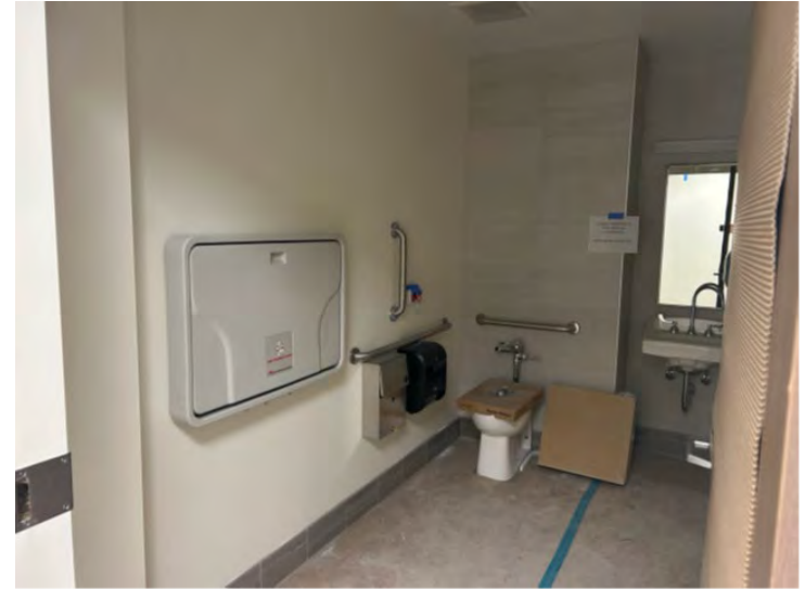
5 th Floor Toilet Room with Accessories
