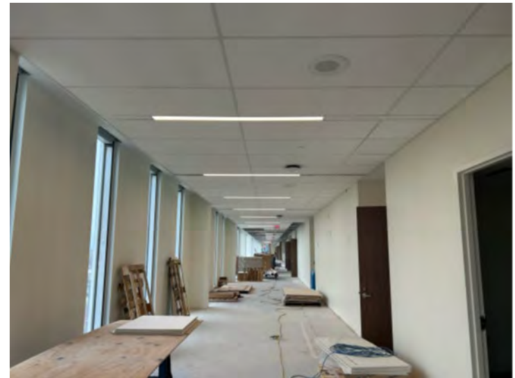
5 th Floor Lobby Completed Ceiling
