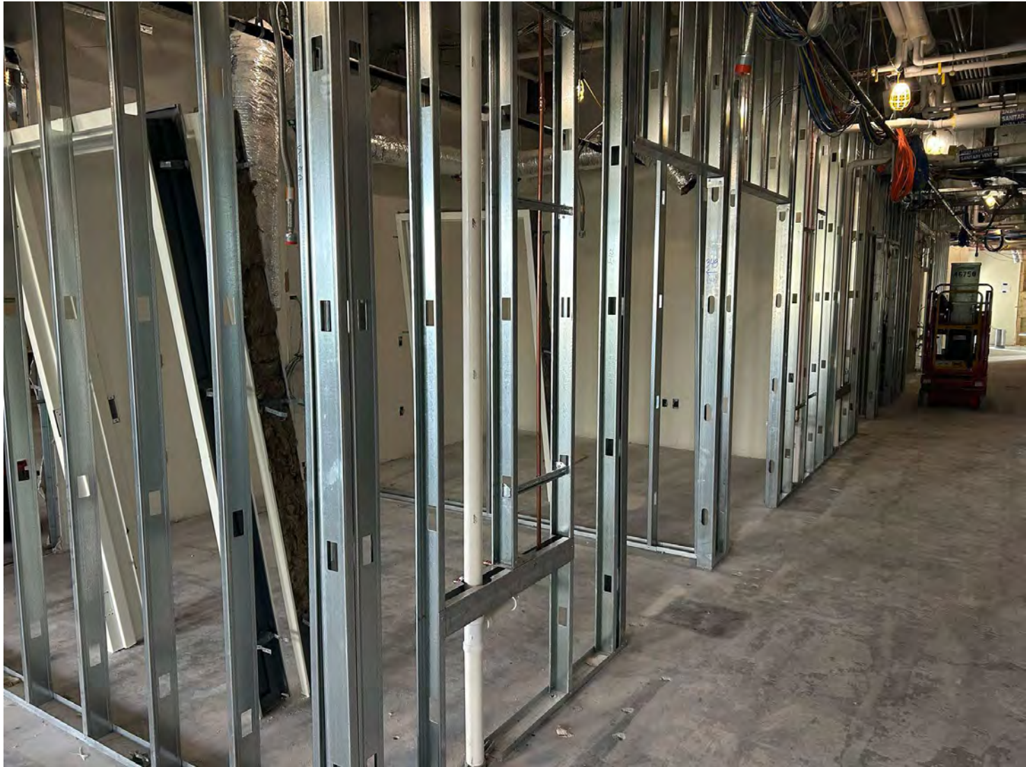
Ground Floor Framing and Door Frames
