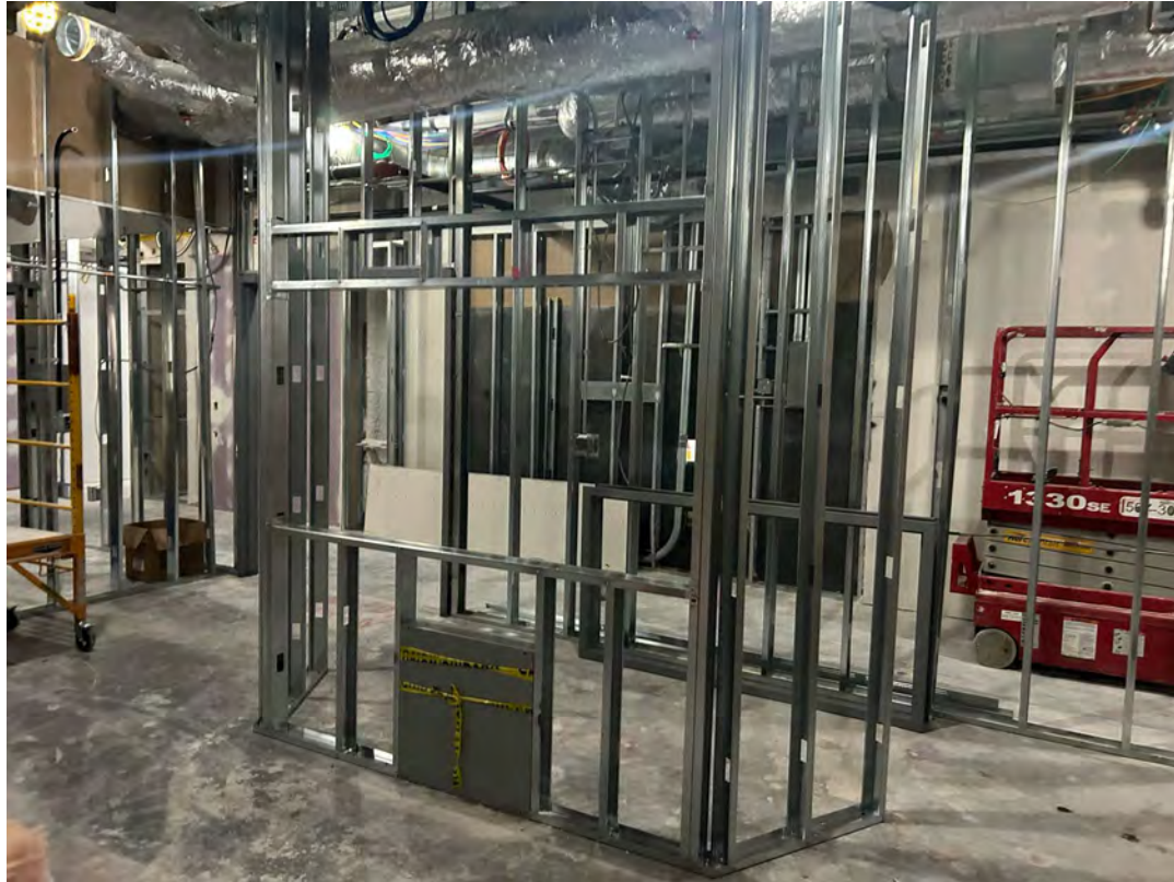
3 rd Floor X-Ray Room In-Wall Rough-In Drywall Installation
