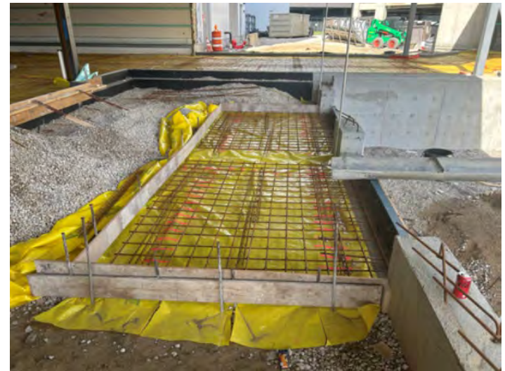
Preparations for Concrete Slab-on-Grade
