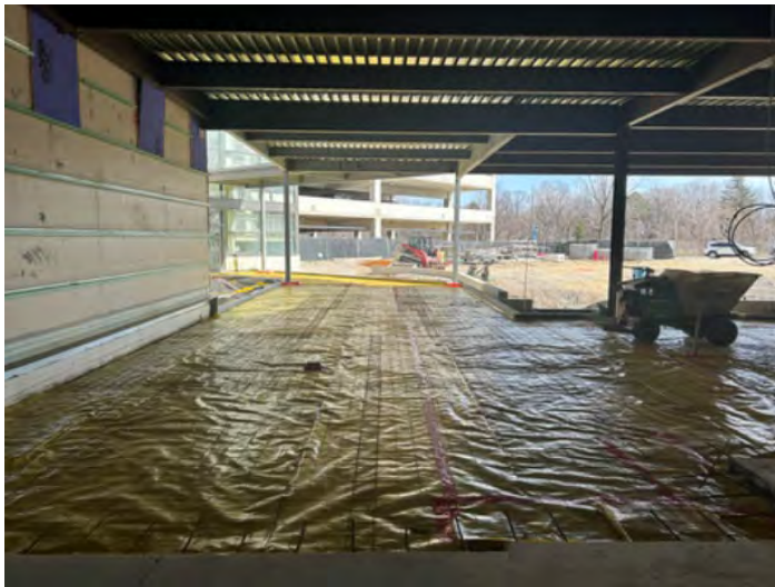
Preparations for Concrete Slab-on-Grade
