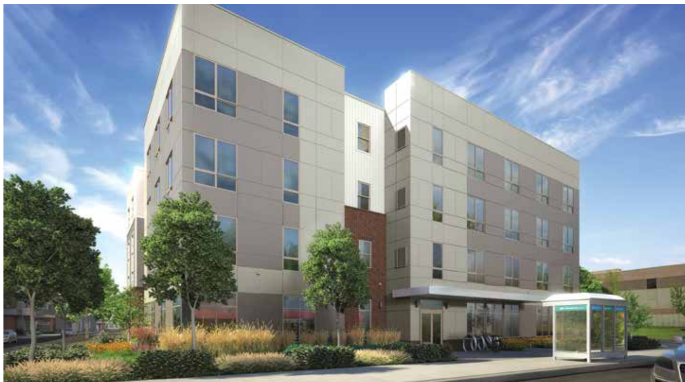
Rendering of the Via Sana building, which will house the MetroHealth Economic Opportunity Center.
